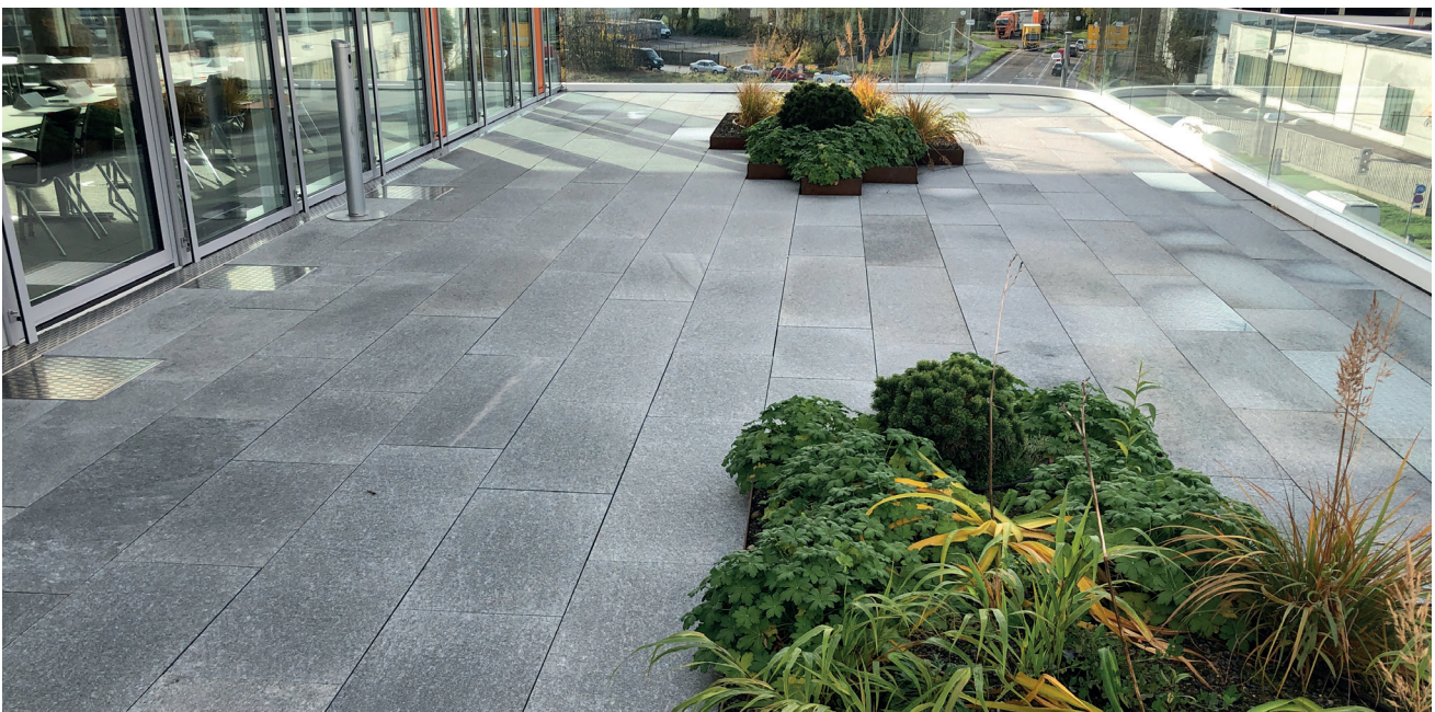
Metal planters and open jointed paving mounted on pedestals
