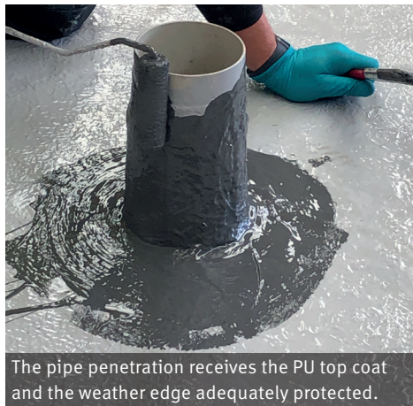
When all the details have received the top coat, the main roof area receives the top coat.
