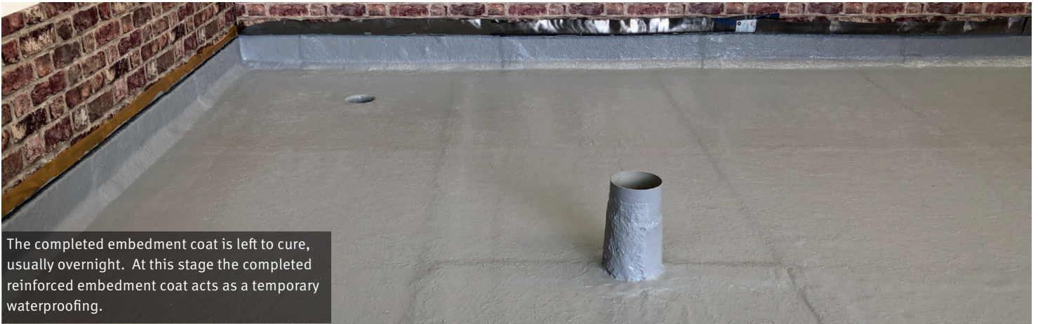
Embedment coat is applied at the details and the glass fibre mat reinforcement embedded.
