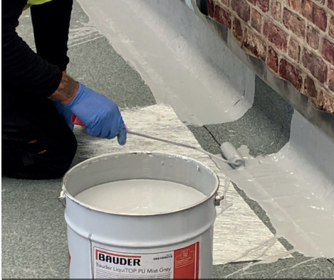
Embedment coat is applied at the details and the glass fibre mat reinforcement embedded.
