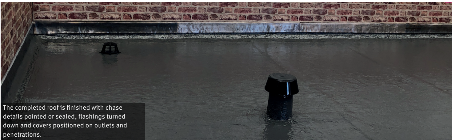
The top coat, seen here in Dark Grey is first applied wet-on-dry to the details.
