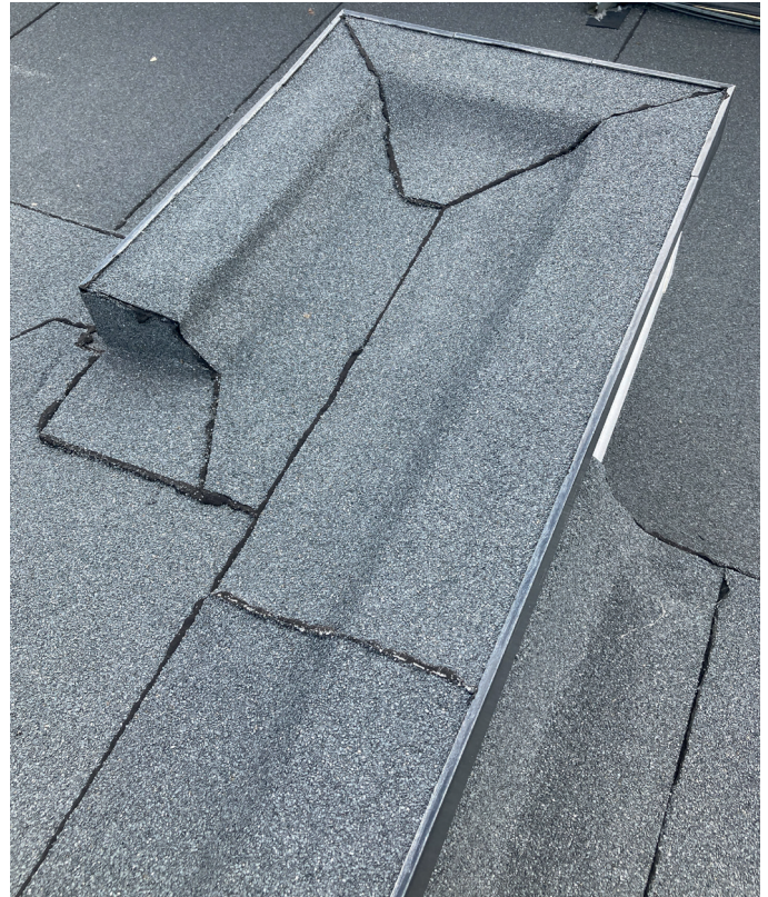
Image showing GRP trim to perimeters
