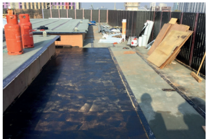
SA Bonding primer installed onto deck
