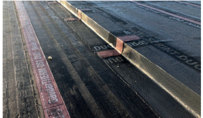
DS 1 DUO installed to field area
