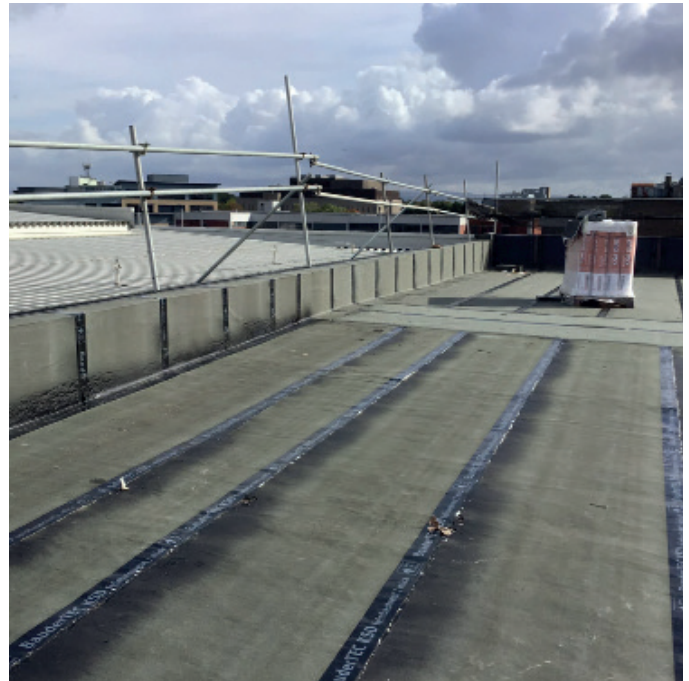
Self-adhesive membrane installed to main field area and upstands.
