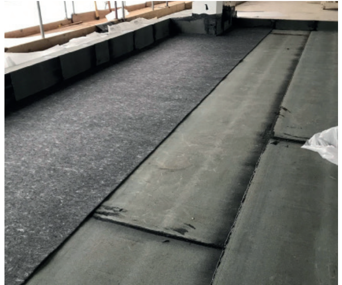
Torch applied AVCL to field area
