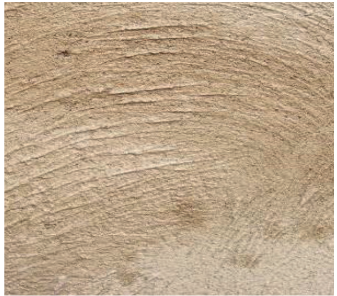
Image displaying concrete deck with a wood float finish
