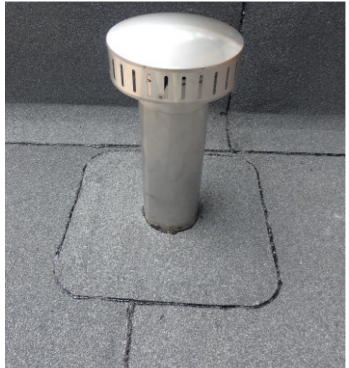
Image displaying SVP cover on bituminous roof
