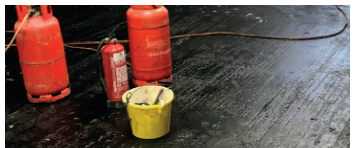
Quick dry primer onto refurb concrete deck
