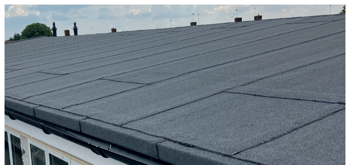
Image of welthed drip to external gutter
