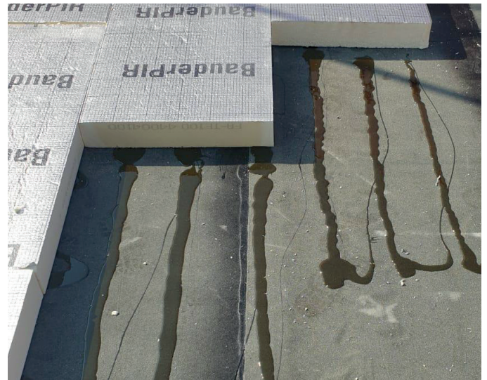
PU Tin adhesive applied in strips
