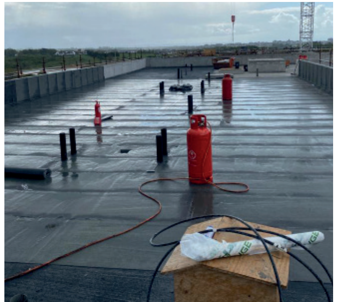
Torch applied AVCL to field area and upstands
