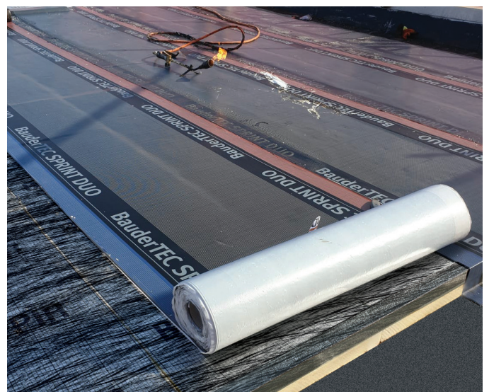
Metal hard edge and insulation facing to be primed prior to installation of the underlayer.
