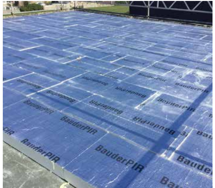
FA-TE flatboard laid off-set and staggered
