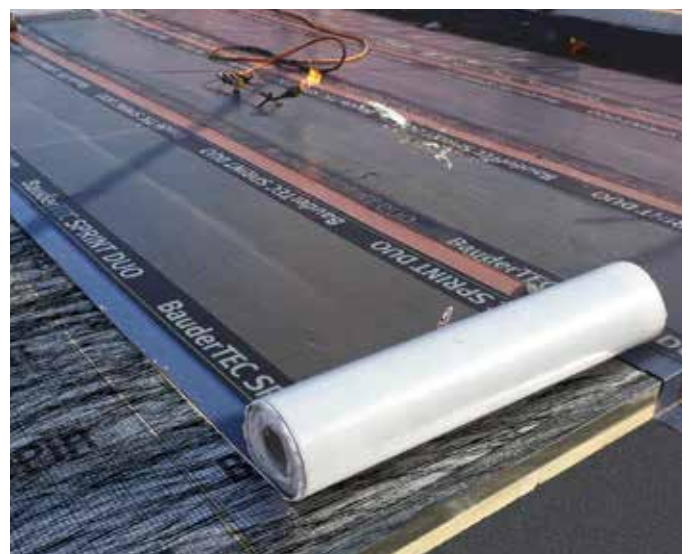
Metal hard edge and insulation facing to be primed prior to installation of the underlayer.
