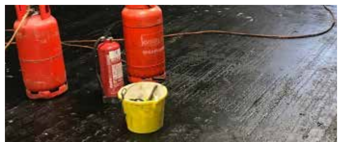
Quick dry primer onto refurb concrete deck
