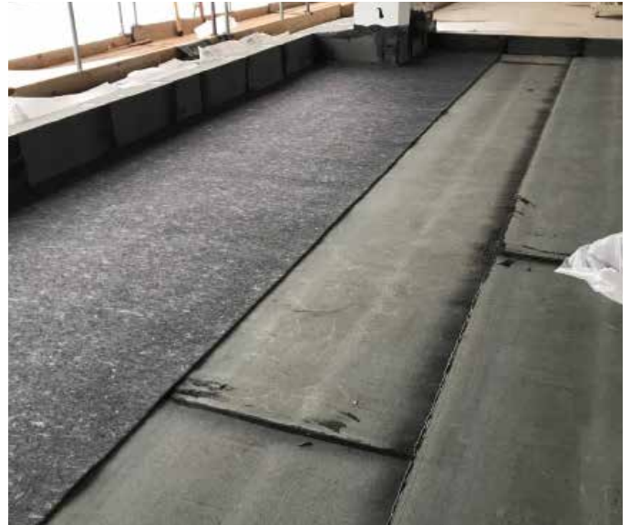
Torch applied AVCL to field area
