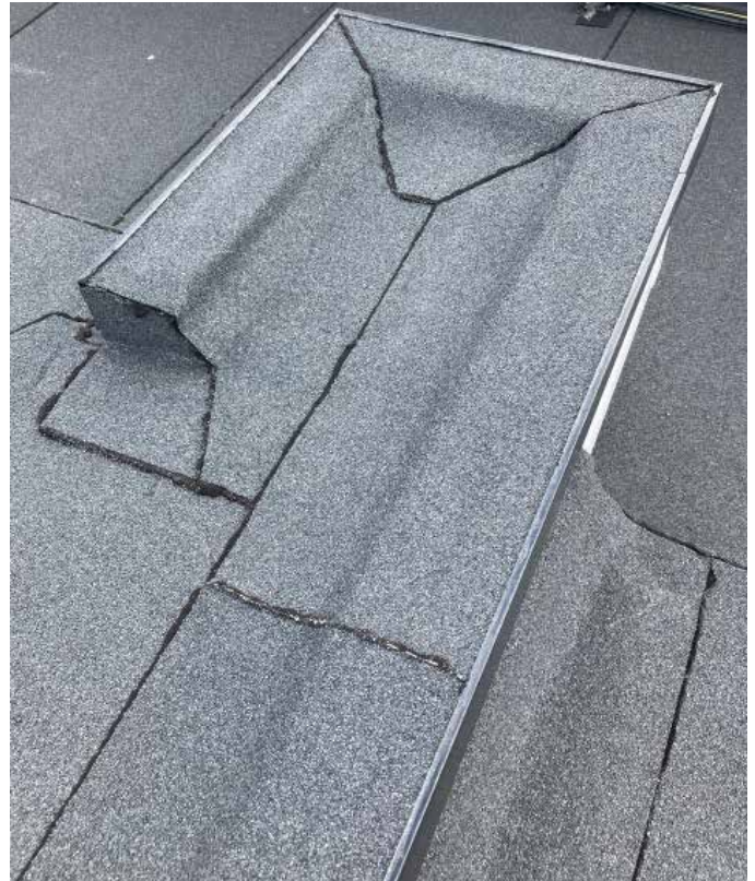
Image showing GRP trim to perimeters
