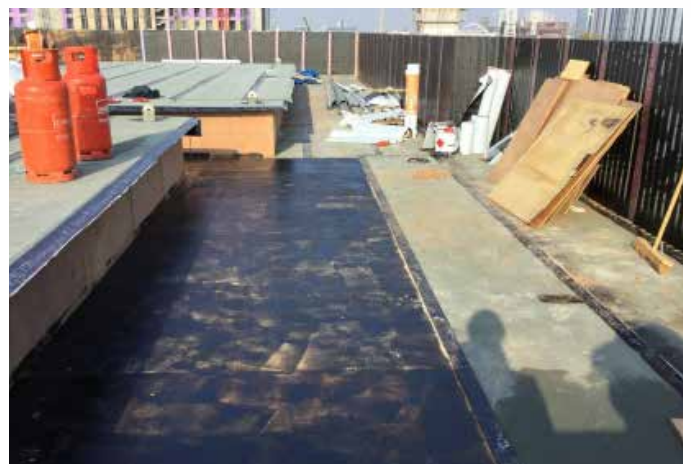
SA Bonding primer installed onto deck
