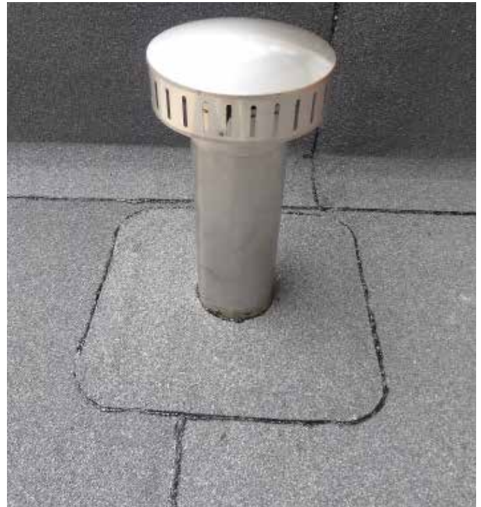
Image displaying SVP cover on bituminous roof
