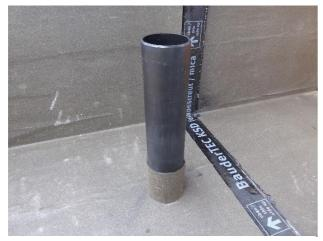
Dress the AVCL up the soil vent pipe a minimum 20mm past the proposed insulation level.
