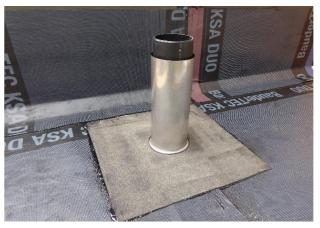
Slide part 1 of the Bauder SVP Cover over the soil vent pipe, and fully bond the integral flange to the underlayer.
