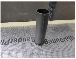
Install the insulation, keeping it as tight as possible to the soil vent pipe.
