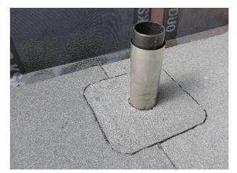
Install the main capsheet, terminating on the flat area at the base of the SVP Cover, and provide a separate capsheet flashing approx. 450mm square to tidy up the detail.
