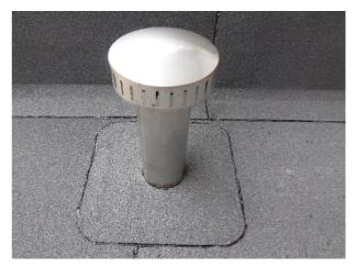
Clean the inside of the soil vent pipe to remove any debris. Slide part 2 of the Bauder SVP Cover over part 1, ensuring that the 'o' ring seals inside the SVP. Install the vented cowl and secure with self-tapping screw.
