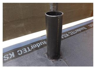
Install the underlayer, ensuring that it laps with the AVCL and provides a watertight seal to the soil vent pipe.
