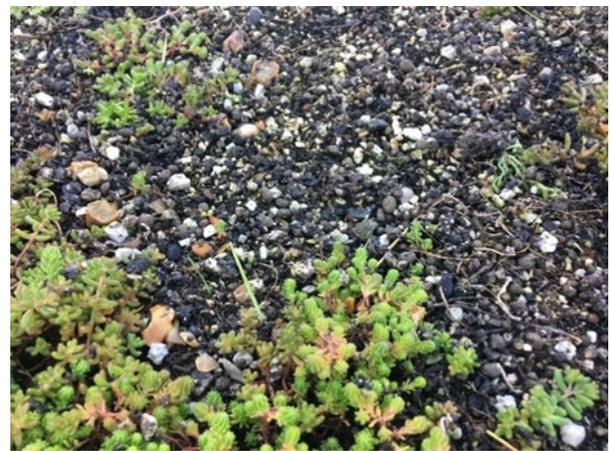
Make sure blankets are butted up tight and joints as neat as possible. Fill all gaps with substrate.
